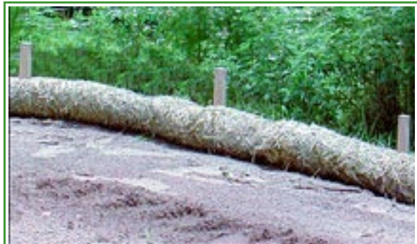
Figure 5. Straw wattle used for erosion control.
