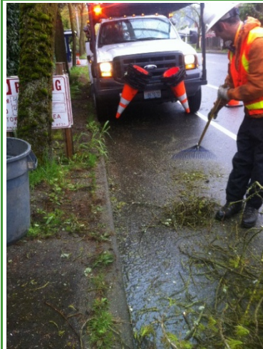
Figure 4. Raking debris out of surface runoff channel.
