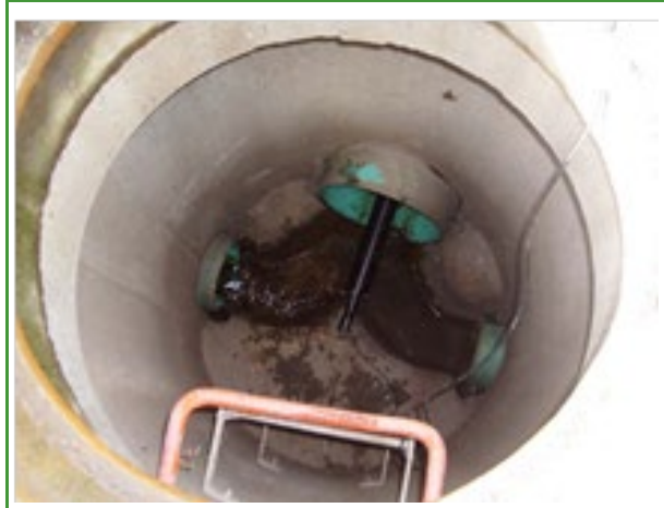
Figure 4. Pipe plug installed prior to catch basin repair work.
