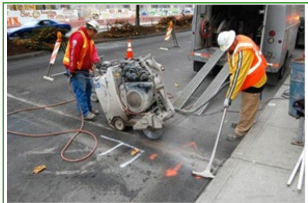
Figure 5. Vacuuming slurry during concrete cutting.
