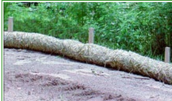
Figure 5. Straw wattle used for erosion control.
