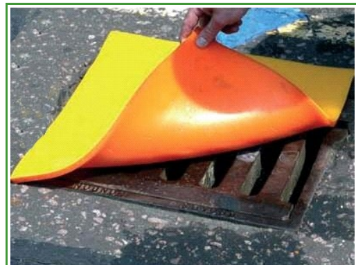
Figure 1. Drain cover used during a pavement striping application.
