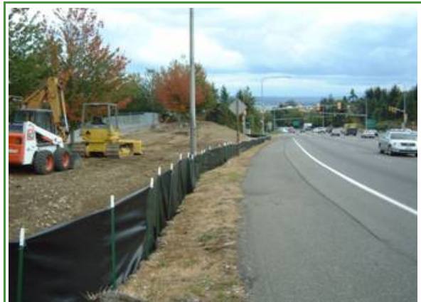
Figure 6. Silt fence used for erosion control.
