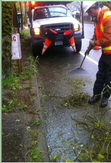
Figure 4. Raking debris out of surface runoff channel.
