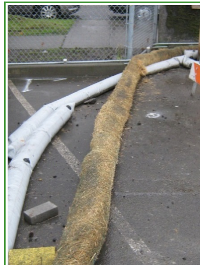
Figure 3. Water-filled barrier dam and straw wattles used for containment.
