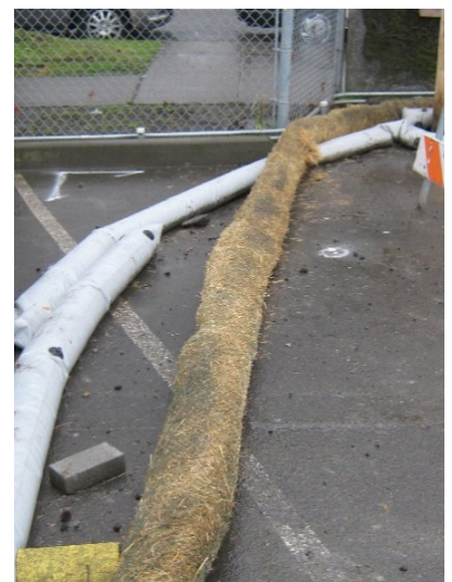
Figure 3. Water bladders and straw wattles used for containment.
