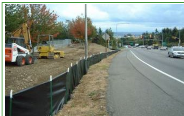
Figure 6. Silt fence used for erosion control.
