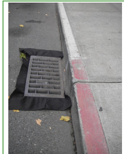
Figure 1. Filter fabric.
