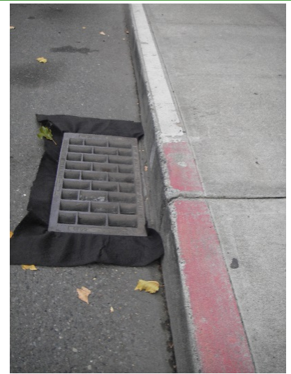
Figure 1. Filter fabric.
