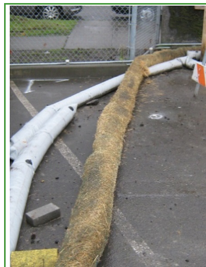
Figure 3. Water-filled barrier dam and straw wattles used for containment.
