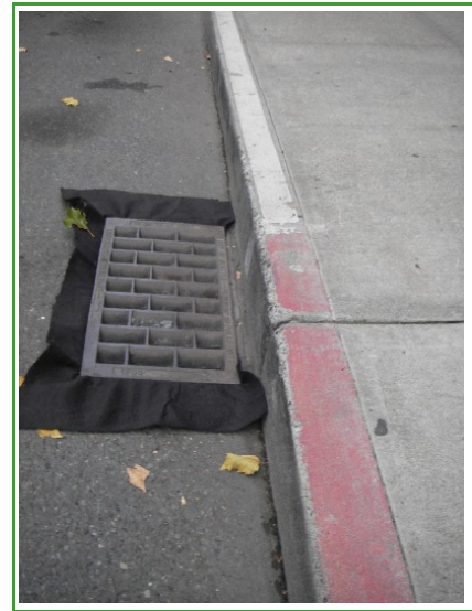
Figure 1. Filter fabric.
