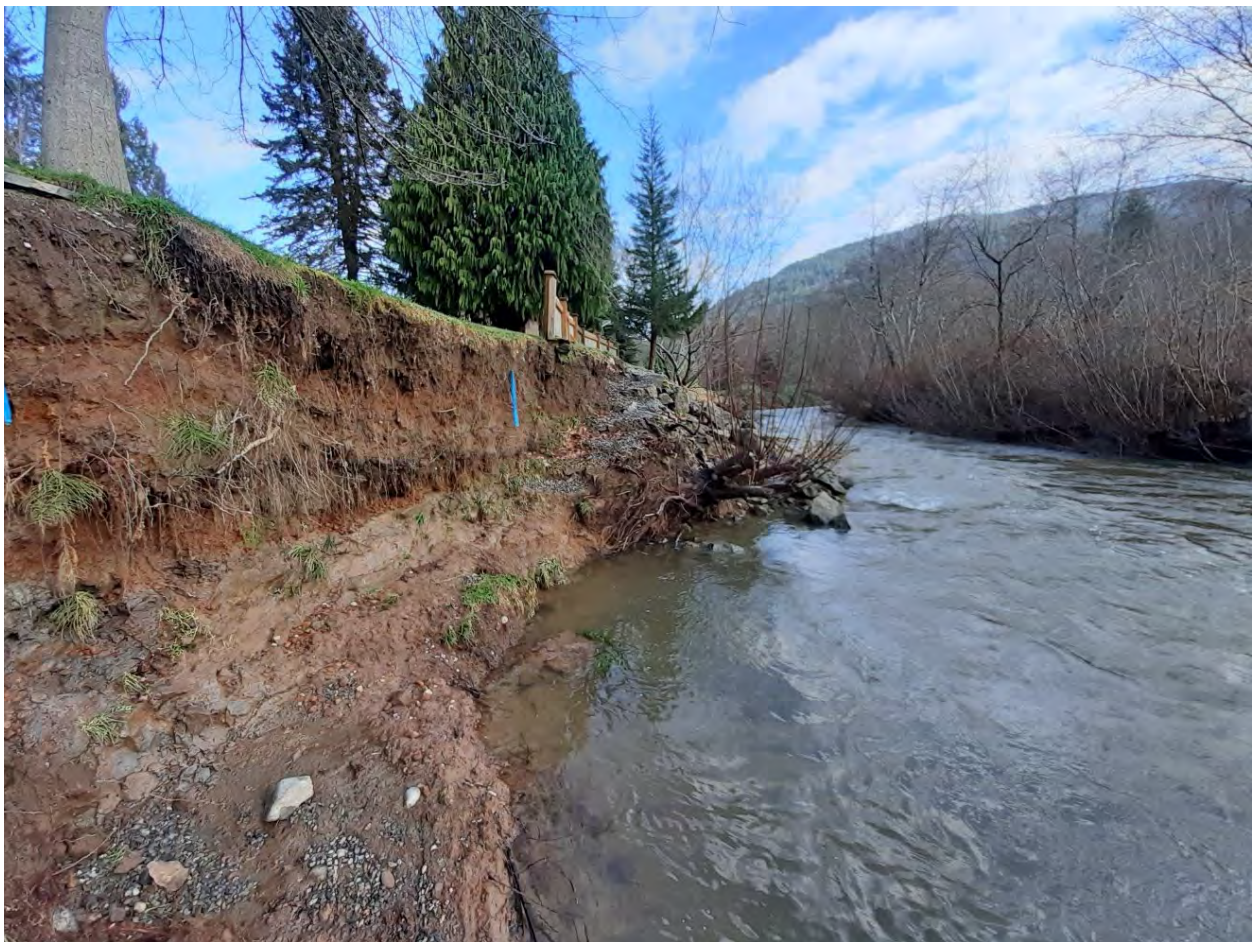
Erosion from Issaquah Creek flooding, January 2021
