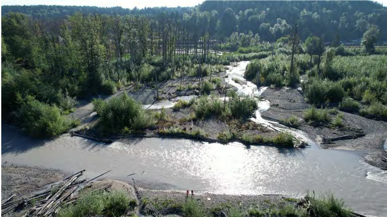
White River Countyline Floodplain Reconnection project, September 2023
